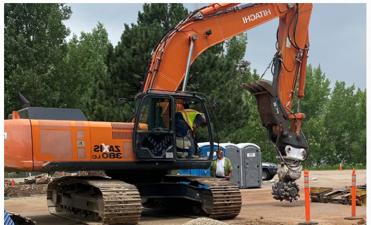
Special equipment allows workers to break through bedrock obstacles.
