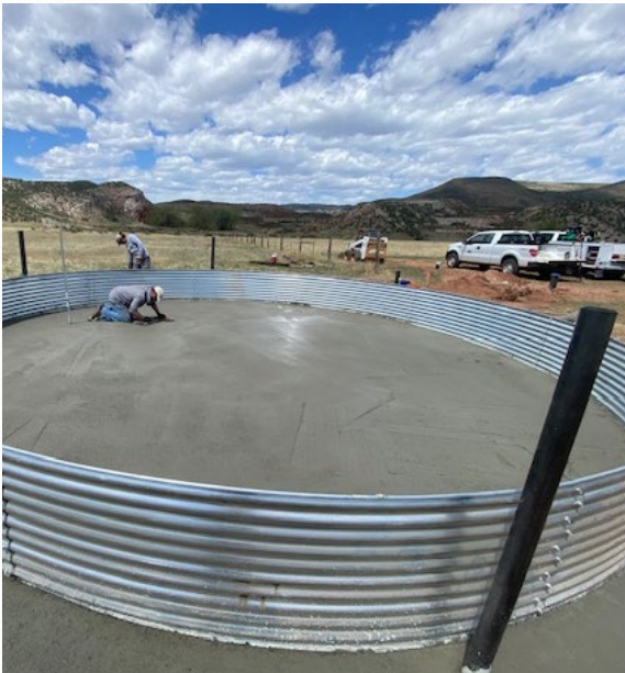
This new water tank will encourage greater grazing distribution to improve native vegetation at Red Mountain Open Space.
