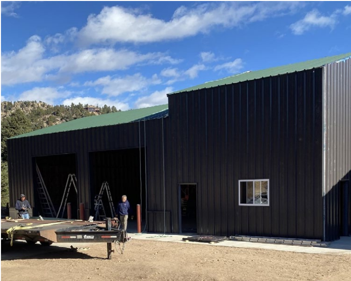
The new maintenance shop at Hermit Park Open Space
